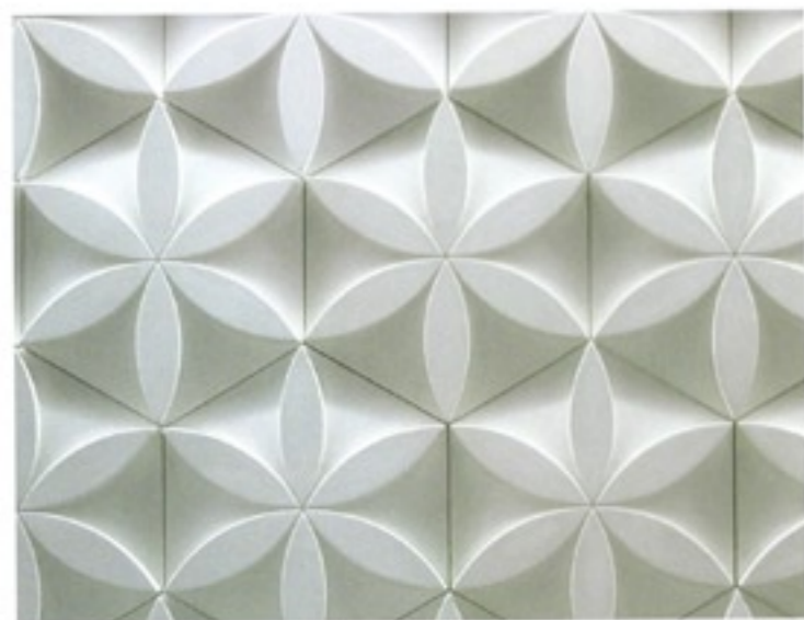
1 The long eastern wall is crafted out of white ceramic 3D hexagonal tiles.
